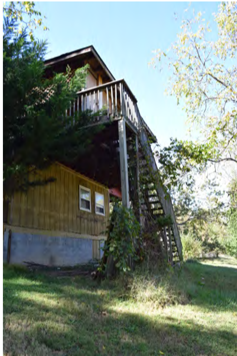
Rear elevation with addition, porch and stair, view to the northwest
