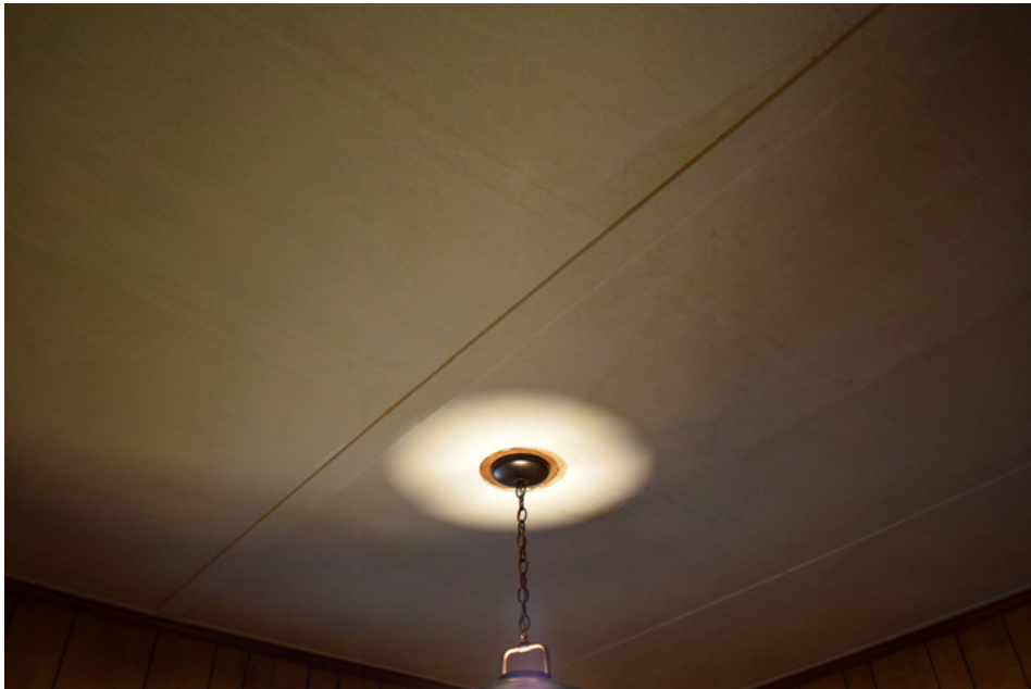
Masonite ceilings remain intact throughout
