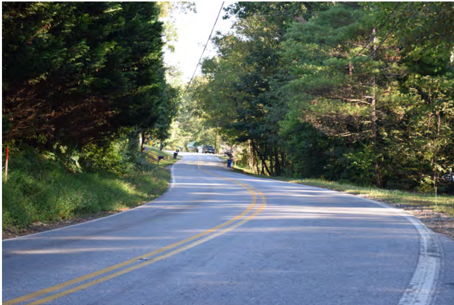
SR 2002 (Riceville Road), view to the north toward Clear Vista Lane
