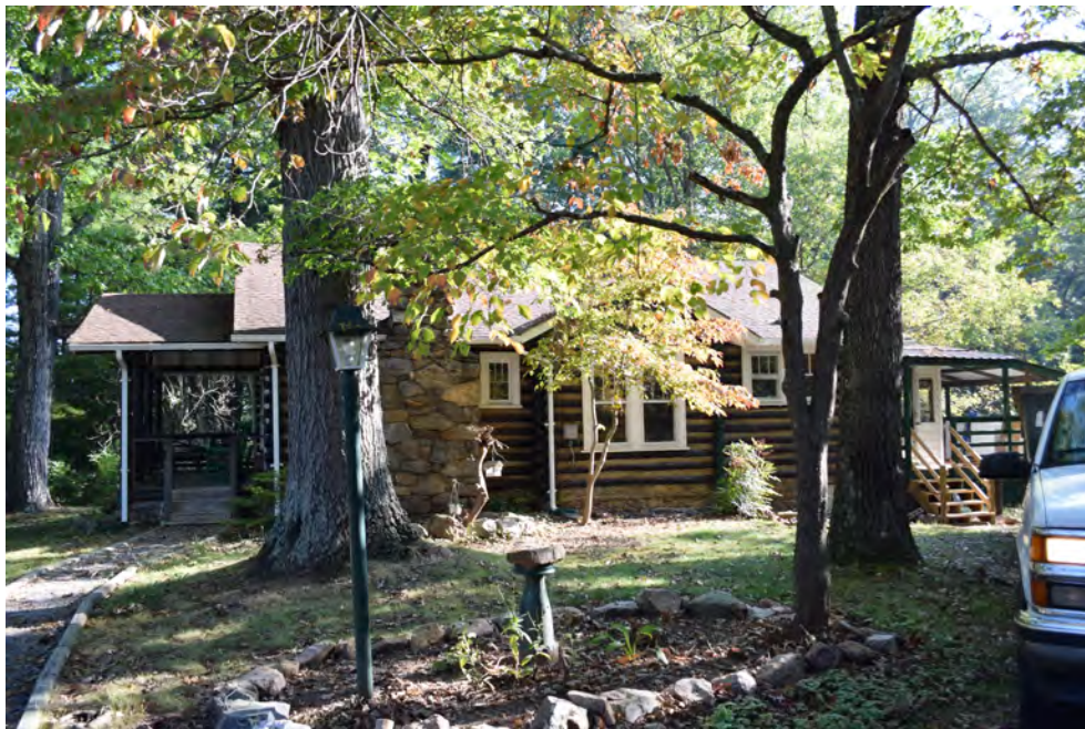
South elevation, view to the north
