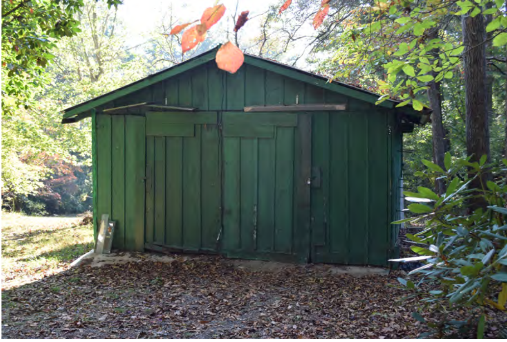
Garage, view to the east
