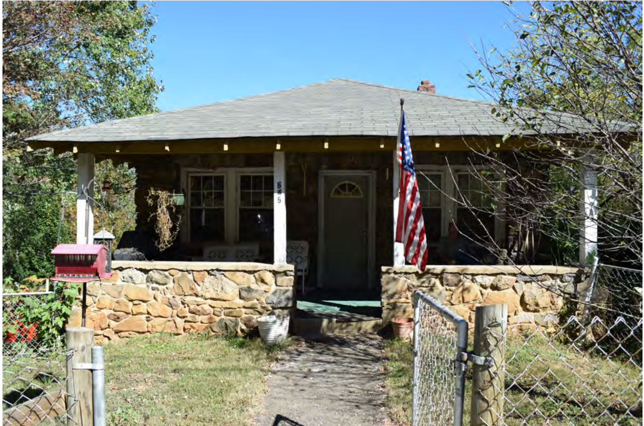
West (front) elevation of the Ella and Horace Emory Matthews House, view to east
