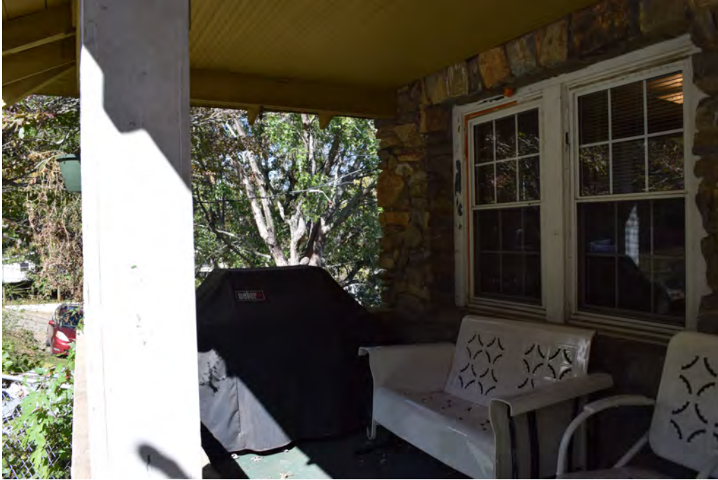
Detail of front porch, view to the northeast
