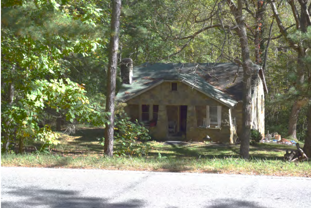
Cole House at 8 R. C. Cole Lane, view to the southeast
