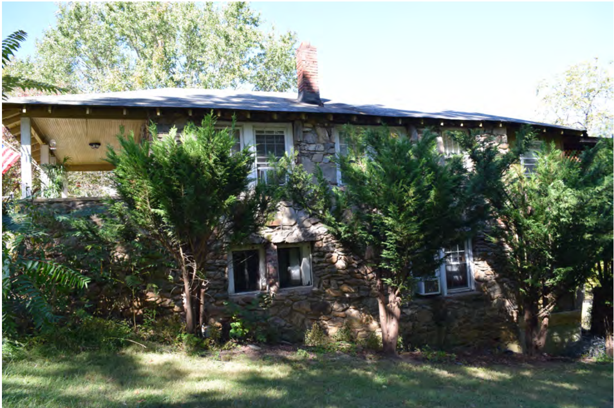
South (side) elevation, view to the north
